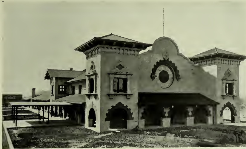
SOUTHERN PACIFIC RAILWAY STATION, SAN ANTONIO, TEXAS. Roofed with Spanish tiles made by the Ludowici-Celadon Company.
